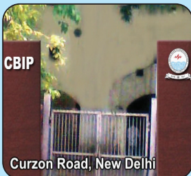
CBIP office at Curzon Road, New Delhi (1952-1980)
