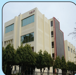
CBIP office at Chanakyapuri, New Delhi (1980 onwards)
